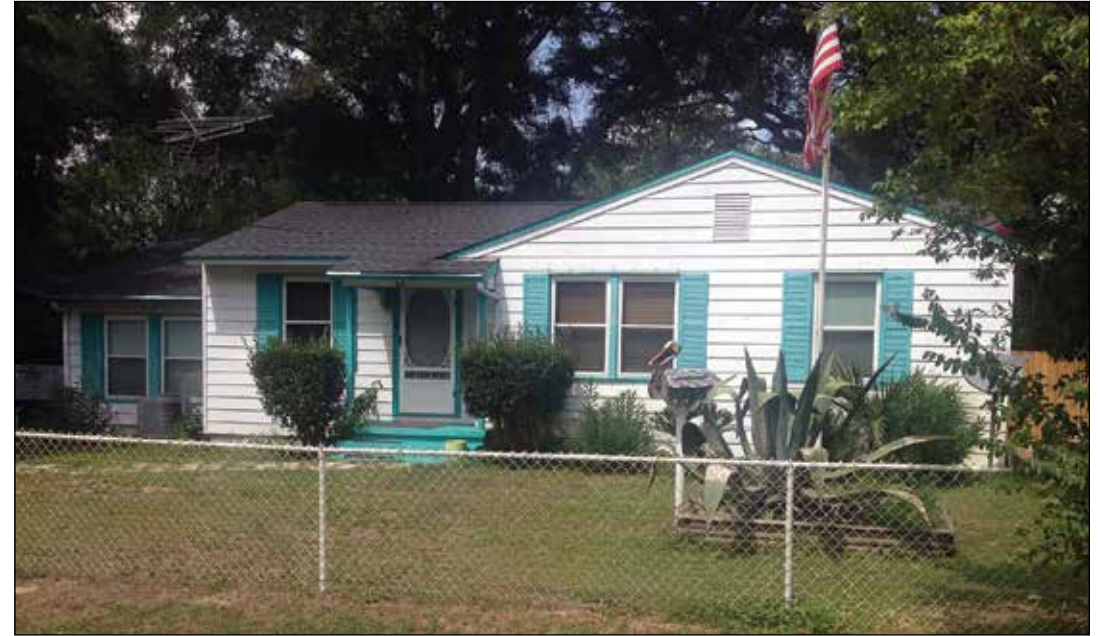
Roof replacement and storm window installation are some of the eligible improvements offered through the CRA Residential Rehab Grant Program.
