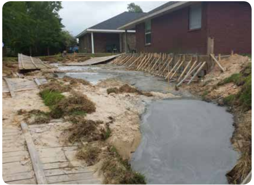
April 2014 flood damage - Newcastle
