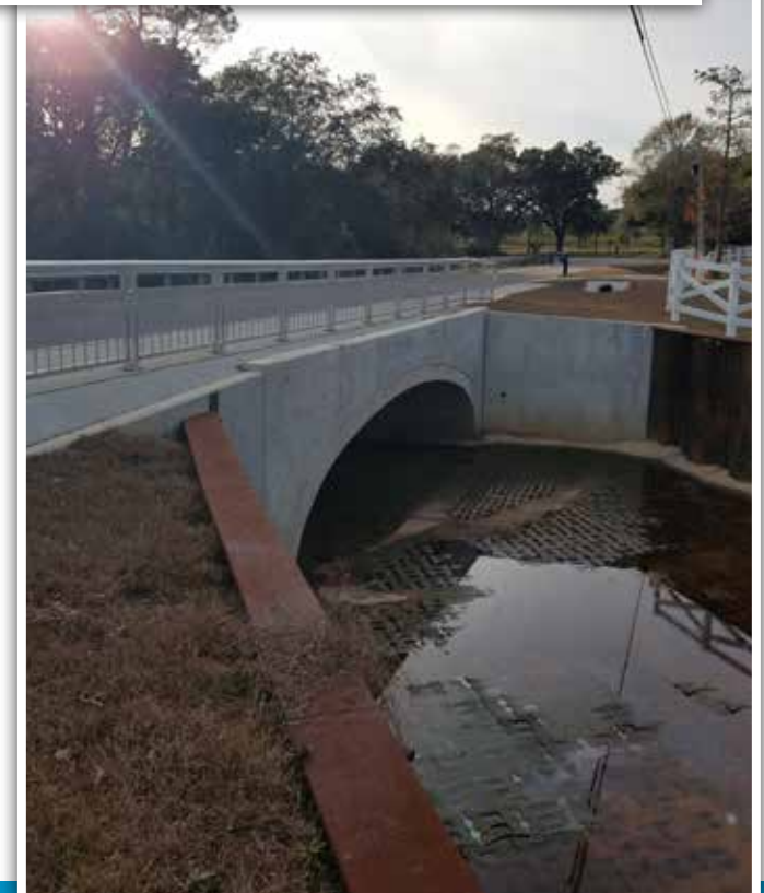
Above and right: The Wilde Lake Boulevard project before and after
