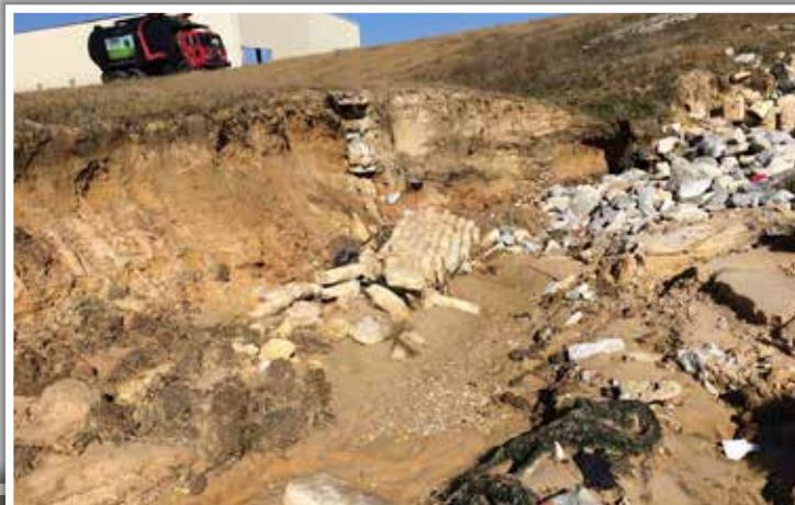
Before and after photos of the Central Conveyance Stormwater Restoration Project
