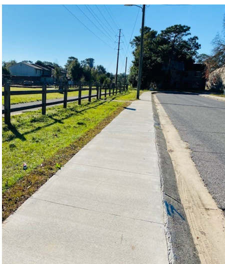
DIEGO CIRCLE SIDEWALK PROJECT
